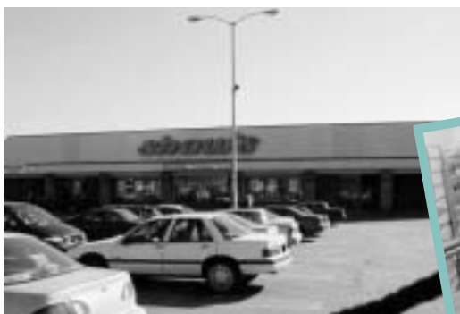
Shaws Markets store at Waymass, Massachusetts, where the first AW-3600AT was installed
